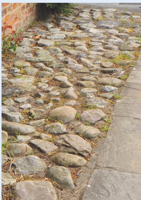
Local brick, cobble and York stone used to good effect.
